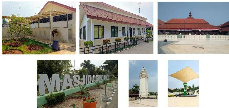
Figure 2. Field observation on the Great Mosque of Old Banten (Masjid Agung Banten Lama)
