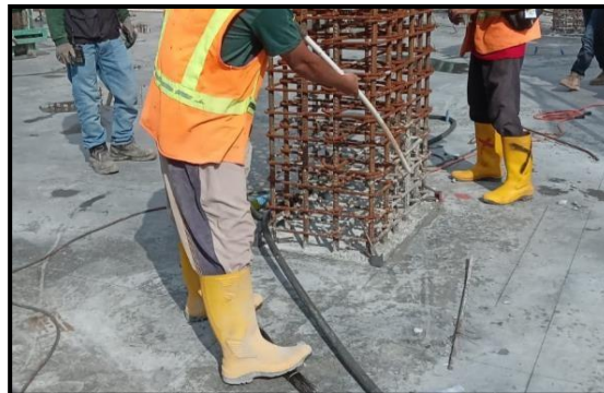
Figure 8. Column Cleaning
