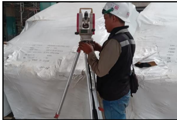
Figure 2. Determination of Column Axis
