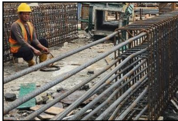
Figure 3. Column Reinforcement Fabrication
