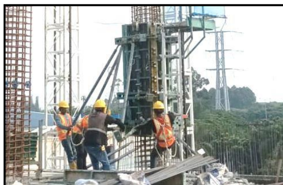
Figure 9. Column Formwork Installation
