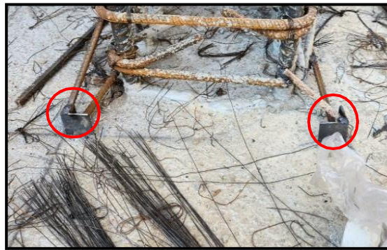
Figure 5. Column Base Installation
