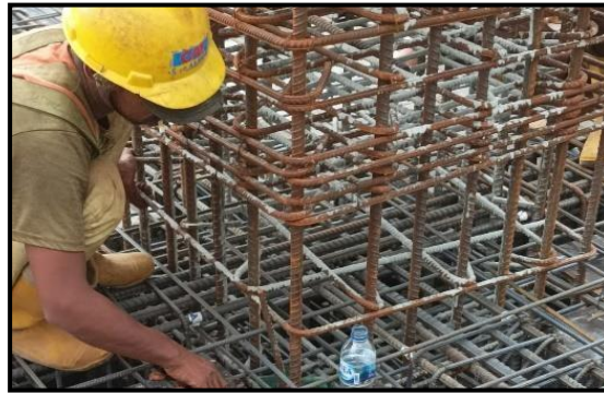
Figure 4. Column Reinforcement Installation
