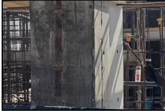
Figure 13. Column Curing
