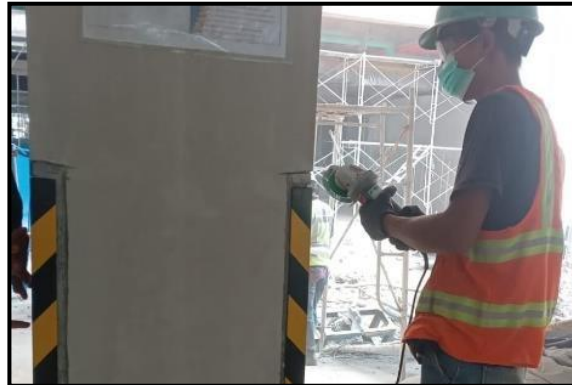
Figure 14. Corner Guard Installation
